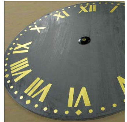
After: original perfectly replicated in GRP.
