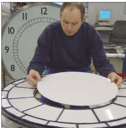
Cast iron skeleton dial being re-glazed with translucent opal acrylic for backlighting.
