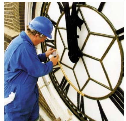
Access to a historic clock tower dial from scaffolding in place for other building work.
