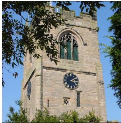
Newly restored church clock dial, cast iron skeleton type with sheet copper backing.
