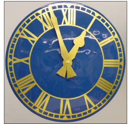
Newly restored dial, hand beaten copper convex with unusual skeleton style numerals and rings.
